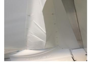
Step 3: Find the first grommet where the body forms a tube. Pull taut and install 6 inches off the sidewall.
