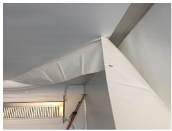
Step 5: Attach the remaining grommets to the ceiling, 3 inches off the sidewall or against the inside edge of the cove mold.
