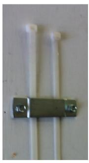
1. Insert 2 of the provided 24" plastic ties through the mounting bracket mounted on the wall
