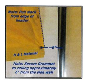
3) <u>Secure outside edges</u>: Permanently secure the remaining grommets between those placed in Step 1 and Step 2. Ensure that there is not excessive slack (over 1/2" sag) between any two of those grommets. Repeat for the other side
