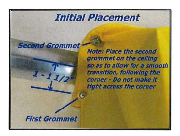
2) Position last grommet: Locate the last grommet along either outside edge. This is the grommet that will be rear-most on the header. After lightly removing the slack from that edge of the header, secure the grommet 6" from the side wall. Note: This location is critical to the efficiency of the tube chute performance as it helps to minimize kinks as the tube chute is aligned with the side wall. Repeat for the other side.
